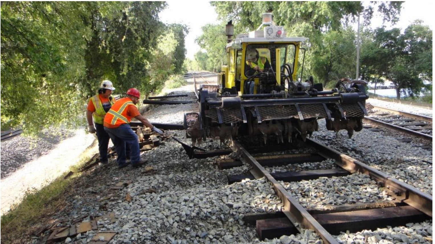
Alan operates the inserter function on the scarifier as Mike F. and Joe guide the tie into place on the Miller Park Siding
