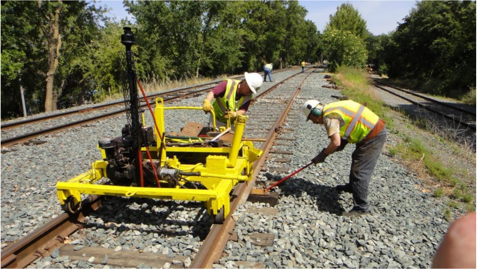
After the ties are tamped, Mike H. employs the rail-lifter as Fred places a tie-plate under the rail.
