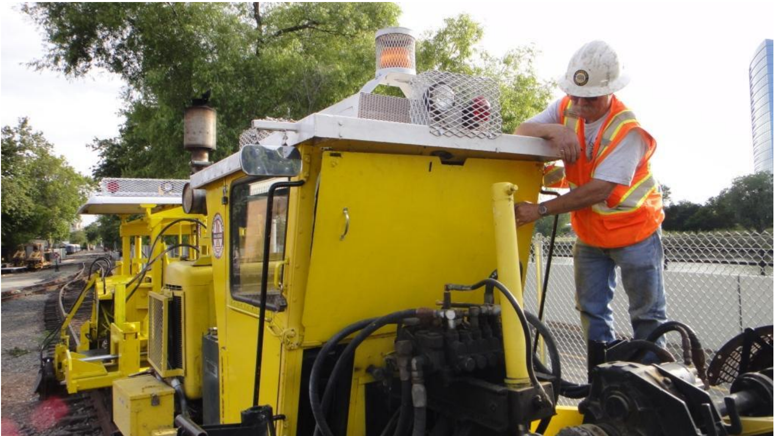
Mike H. lowers the shields on the scarifier.
