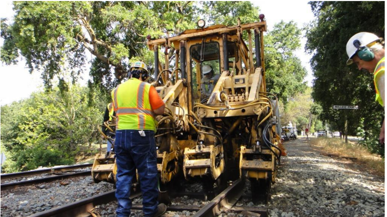
Mike F. guides Steve in tamping-up the new ties.
