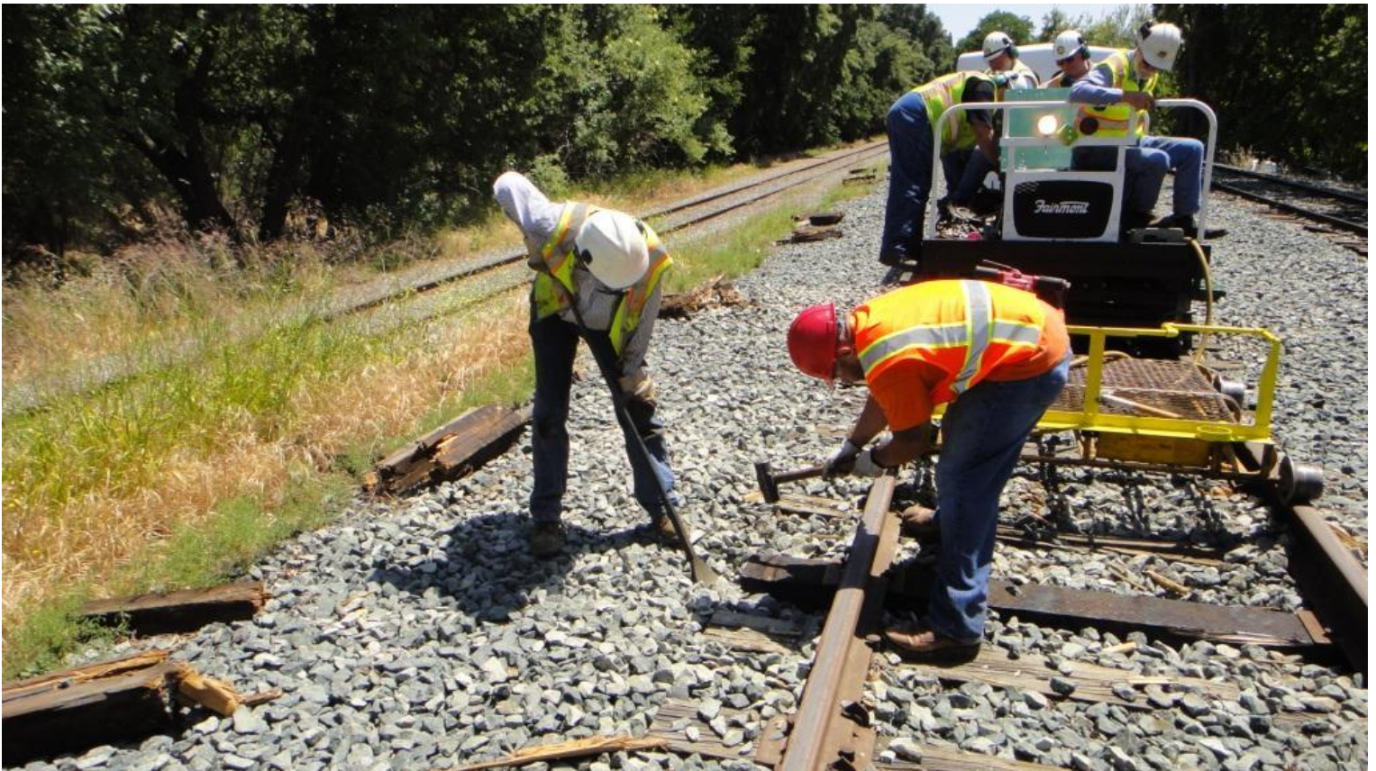
Meanwhile, back at the work-site, Steve nips up the tie as Joe sets spikes
