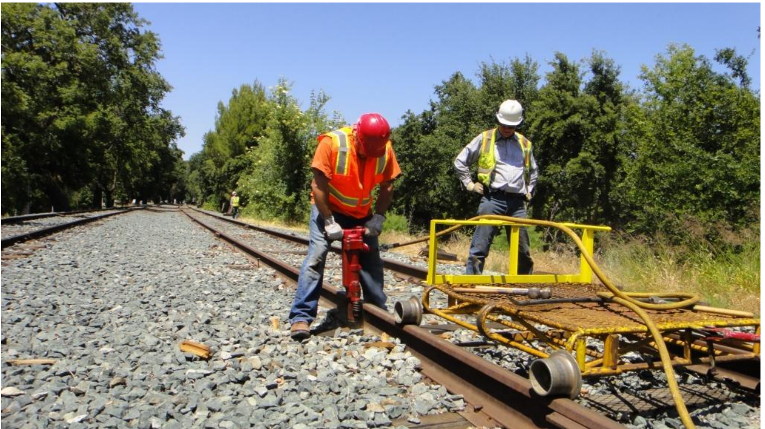
Now it's Joe's turn at the pneumatic spiker.
