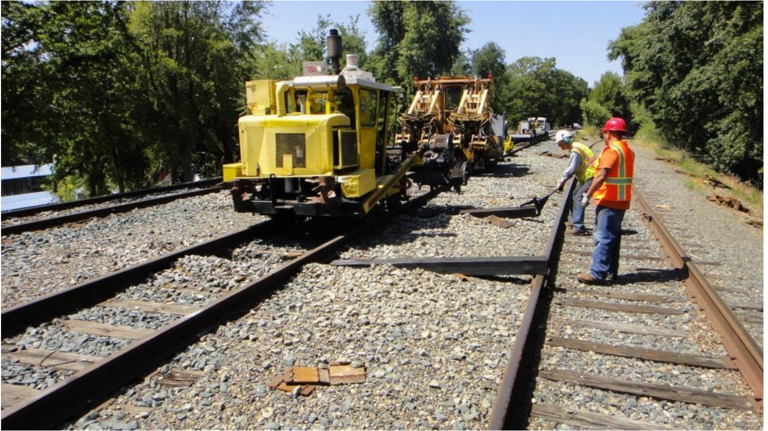
As we were ahead of schedule, we decided to insert more ties in the afternoon. Steve guides a new tie into position.
