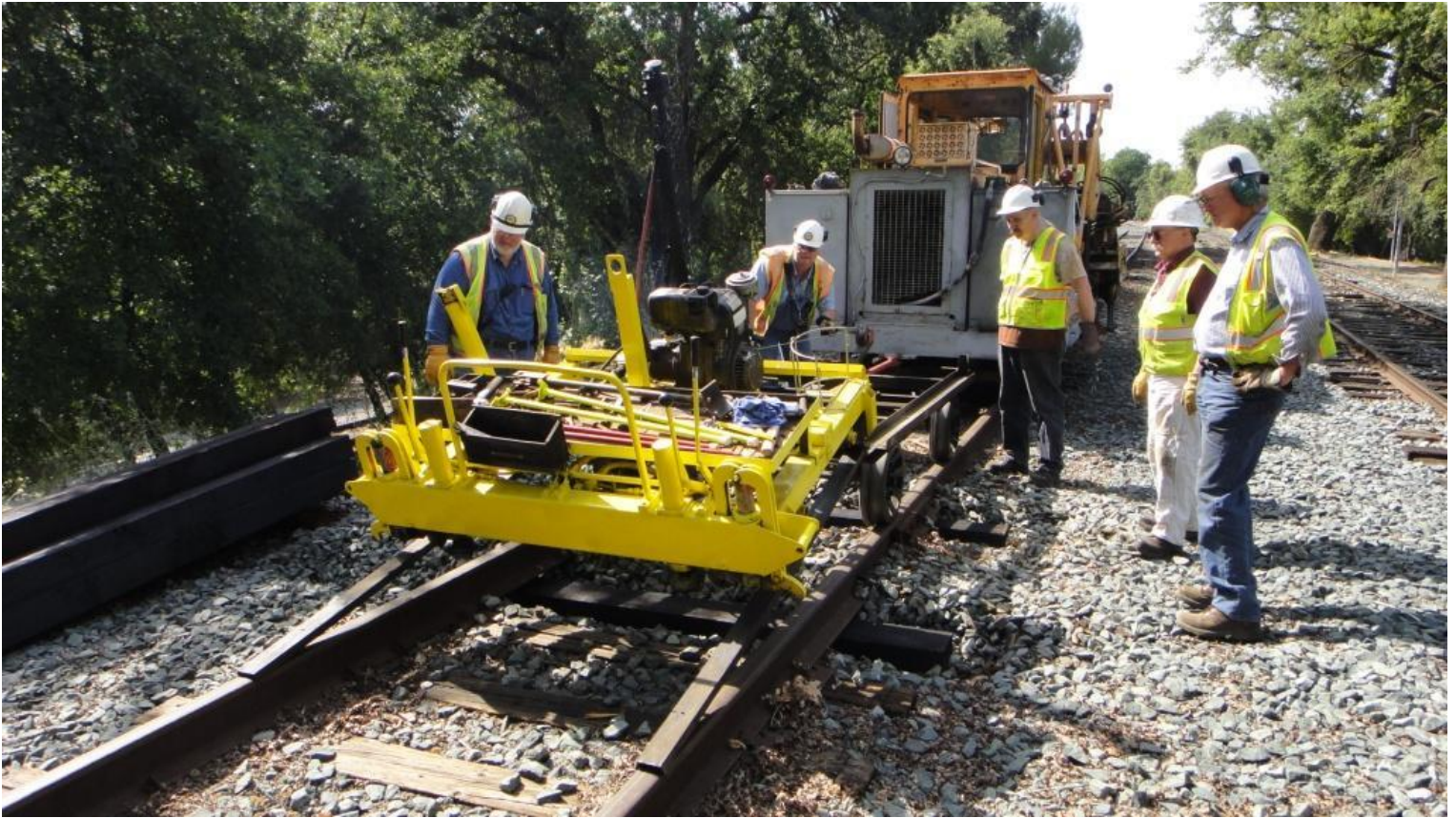
Frank W., Chris, Fred, Mike H., and Steve deploy the rail-lifter.
