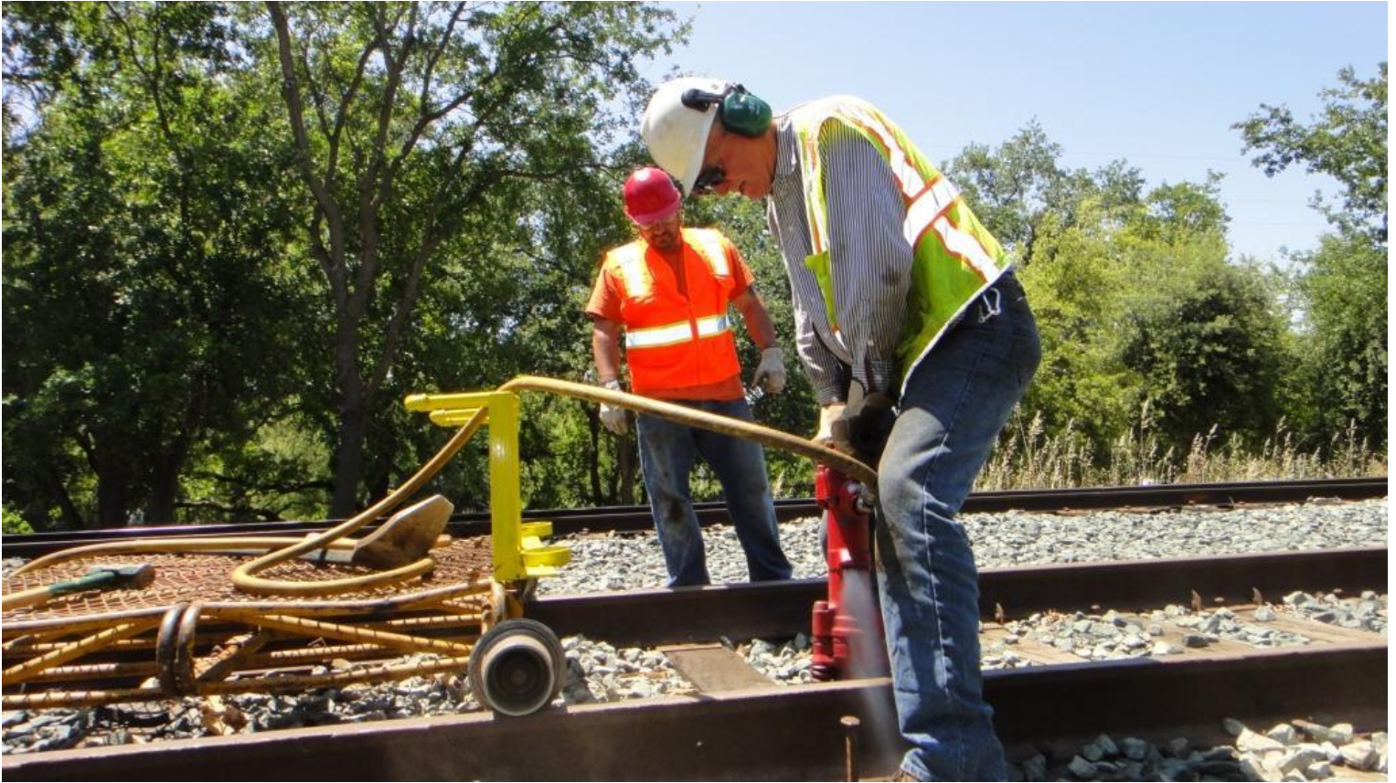
Steve uses the pneumatic spiker to drive spikes into the new ties.
